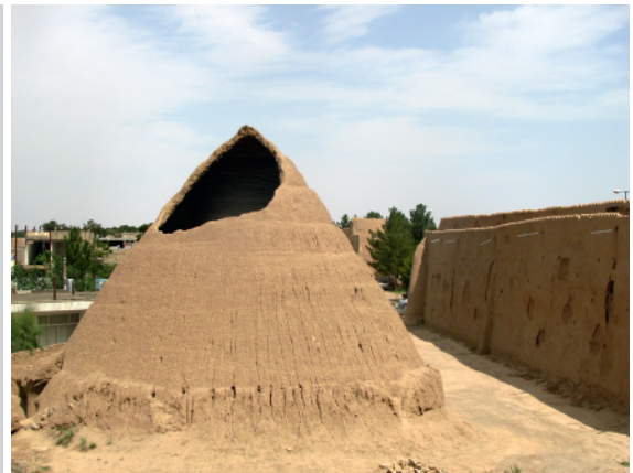
Figure 4. Remains of the Icehouses with shade walls near Sabz-e-Var. [Author]
