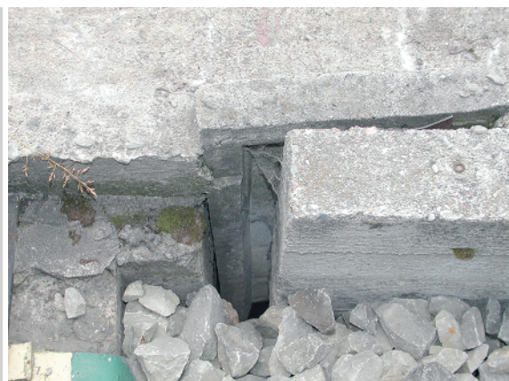
Figure 8. Gap at contact of an approach continuous footing and an oil tank wall
