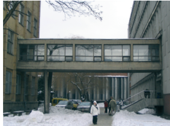
Figure 3. The elevated walkway between the two Faculties
