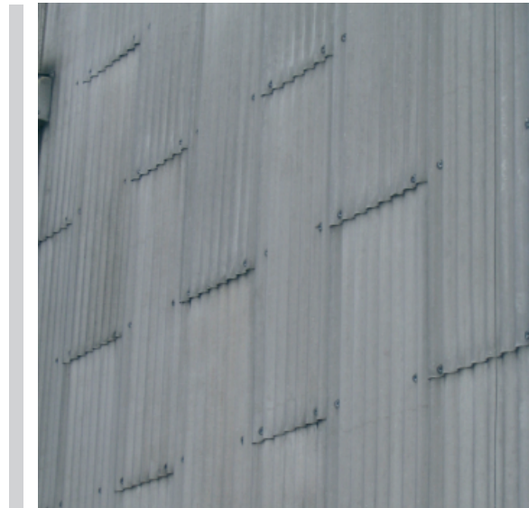
Figure 12. A good spot for the introduction of a new material
