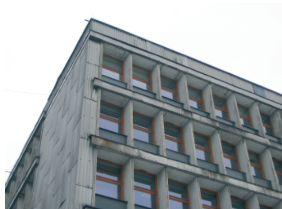
Figure 4 The regularity of ribs and windows
