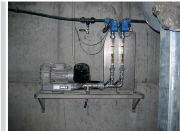
**Figure 6.** Air pump used in a large agricultural biogas plant
