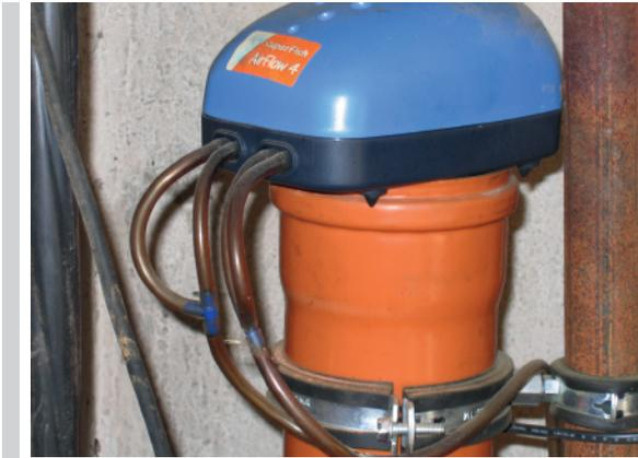
**Figure 5.** Aquarium pump supplying air to oxidize hydrogen sulfide in biogas
