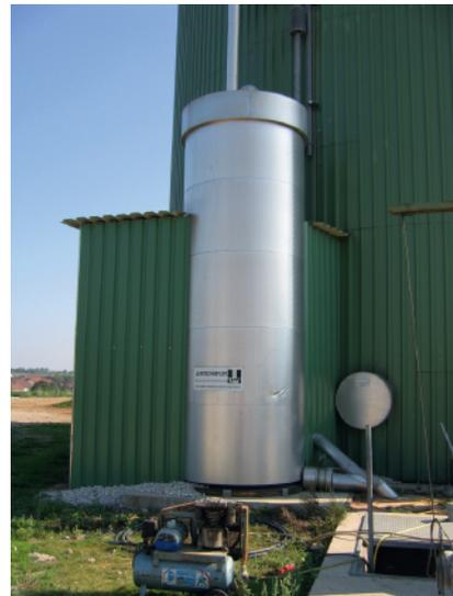
**Figure 9.** Installation for biological removal of hydrogen sulfide in a biogas plant using bird droppings and corn silage in digestion process
