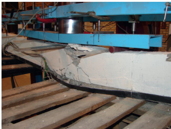
Figure 4. Failure of beam II-1
