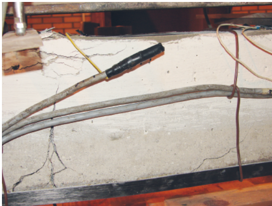
Figure 12. Failure of beam III-2
