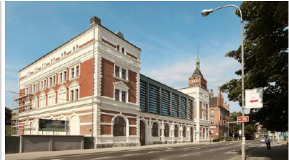
Figure 2. View of the building from the Wrocławska Street
