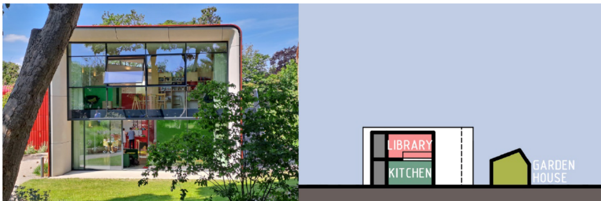
Figure 3. Maggie’s Centre at the Royal Marsden, London – view of one of the elevations and a schematic cross-section through the building. Photo by Rafał Strojny. Drawings elaborated by the authors from online material available at the AB Rogers Design office. Source: https://www.abrogers.com/portfolio/maggies-at-the-royal-marsden/
