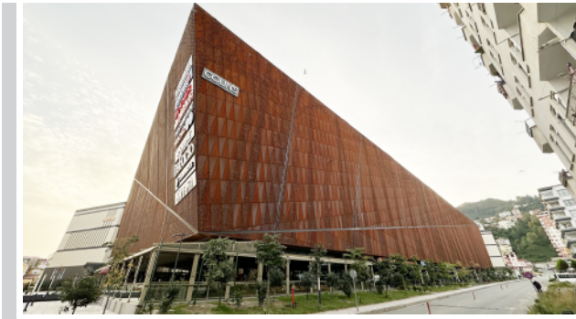
Figure 6. Rize Şimal shopping mall exterior [Source: Authors]
