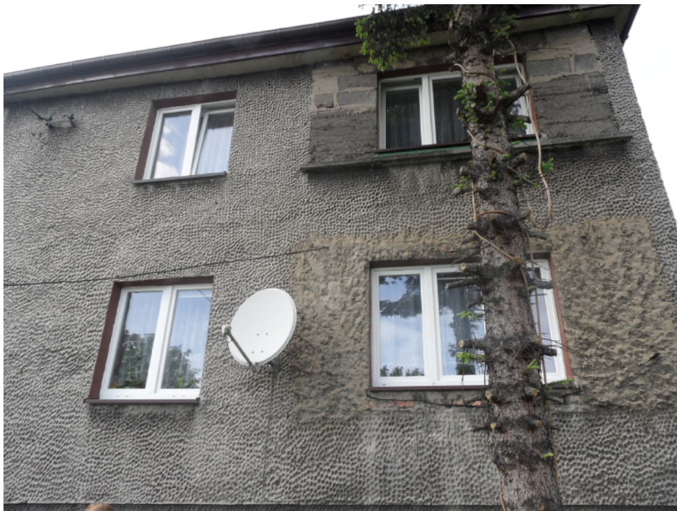
Figure 6. General view of the southern wall of the building
