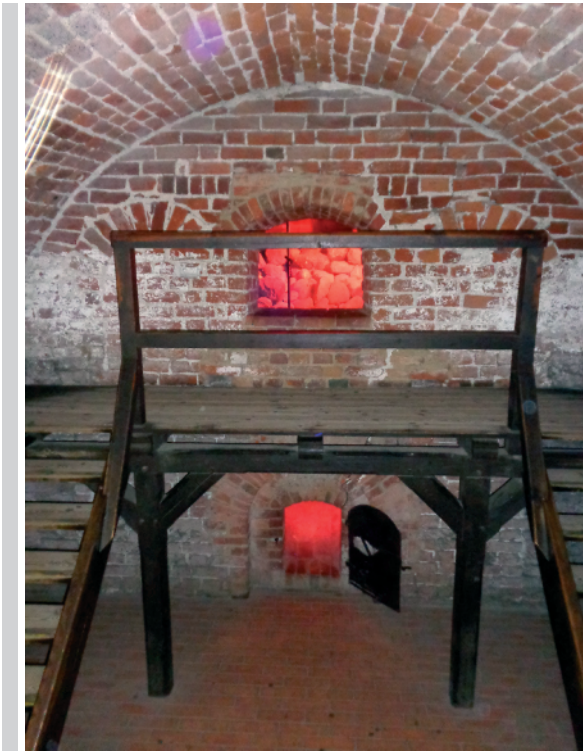
Figure 4. Malbork, Poland, Middle Castle. Heating stove built to heat the Great Refectory, 14 th century: A visible furnace opening at the bottom, an accumulation chamber filled with huge stones at the top. The author's photograph of 2018
