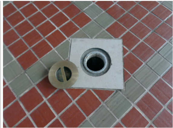
Figure 5. Malbork, Poland, Middle Castle. Great Refectory, 14 th century: One of the 36 openings supplying hot air from the accumulation chamber of the stove located below. The author's photograph of 2018
