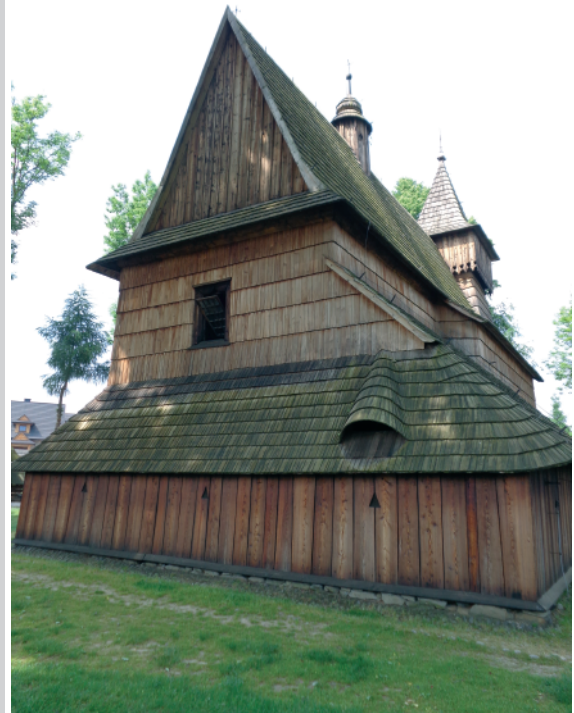
Figure 2. Dębno, Poland, St. Michael the Archangel Church, 2 nd half of the 15 th century: Timbered arcades surrounded all church walls, forming a thermal buffer. The author's photograph of 2015
