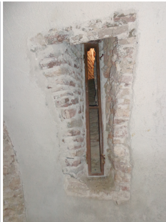
Figure 7. Czorsztyn, Poland, Upper Castle. A ventilation opening in the form of a slot window in the cellar of the Upper Castle, 14 th century. The author's photograph of 2015
