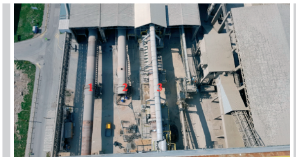
Figure 1. Rotary kilns (top view) (1. One of the three old rotary kilns – currently out of service, intended for demolition; 2. One of the three old rotary kilns – currently being demolished; 3. New rotary kiln)
