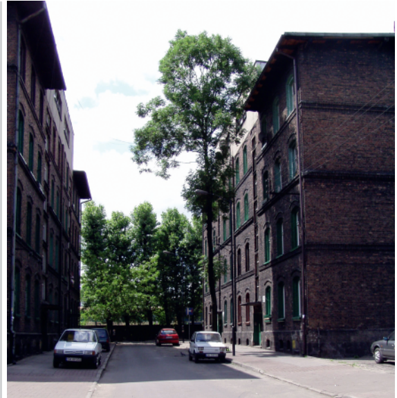
Figure 4. Quarter of workers' buildings in the urban quarter of Katowice Załęże
