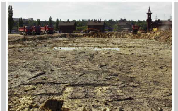
Figure 11. A view of a typical system of clays in the gout of a large building excavation with extremely diverse proprieties, simultaneous drying – the nearer zone and irrigation – the background
