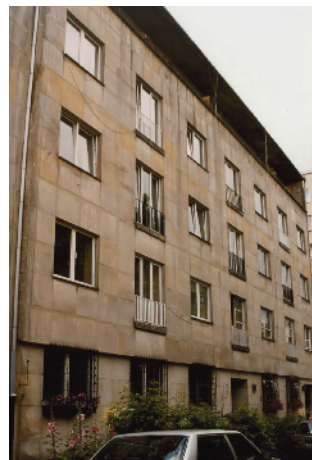
Figure 5. Warsaw, tenement house at Konopnickiej 5 (B. Pniewski, 1936-1938) – east side – façade
