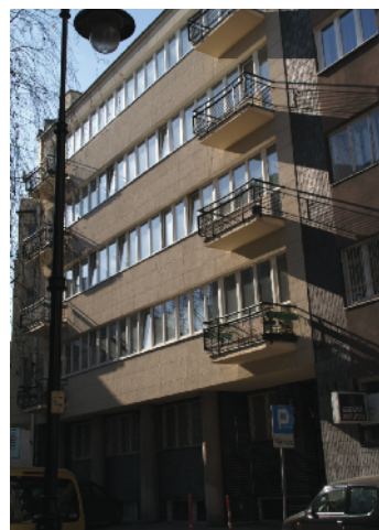
Figure 10. Warsaw, tenement house at Jaworzyńska 6 (H. and S. Syrkus, 1937-1938) – south side – façade
