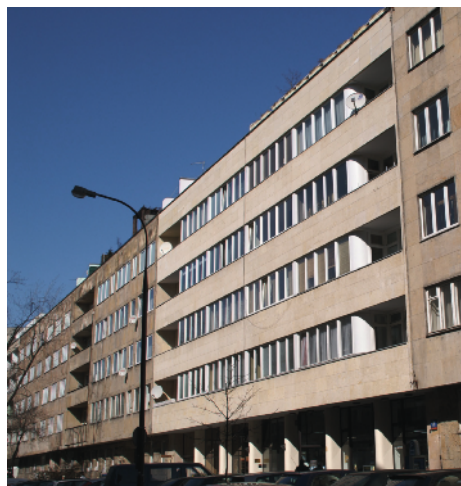
Figure 4. Warsaw, houses at Wiejska street no.: 14 (W. Weker 1935-1938), 16 (L. Korngold 1936-1937), 18 (Z. Mączyński, 1936-1937) – west façades
