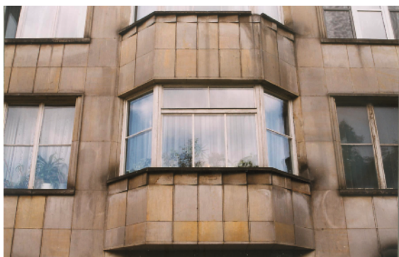
Figure 2. Warsaw, tenement house at Konopnickiej 3 (J. Gelbard, R. Sigalin, 1936-1937) – stone overlay on façade
