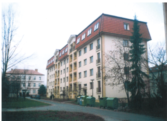
Figure 2. Well done realization of mansard extension in Hranice na Moravě
