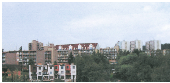
Figure 3. Complex of blocks of flats with sporadic realization of saddle roof extension
