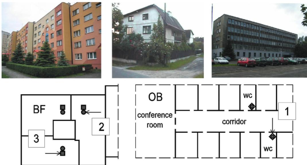
**Figure 2.** View of tested buildings (from the left © block of flats - BF, detached houses – DH and office buildings – OB). Notations: 1- individual ventilation ducts, 2 – collective ventilation ducts, 3 – gas pass ducts
