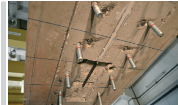
Figure 2. CFRP strip mounted in the groove
