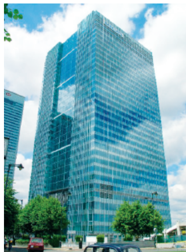
Figure 2. Barclays Bank Head Office, London, UK (photo by Simon Judd)
