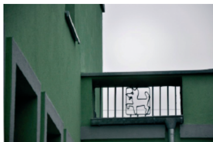
Figure 10. A detail of a terrace banister, made according to a catalogue edited in 1955, Poznań, Nursery School, Trzemeszeńska Street, Poznań (phot. TBB)
