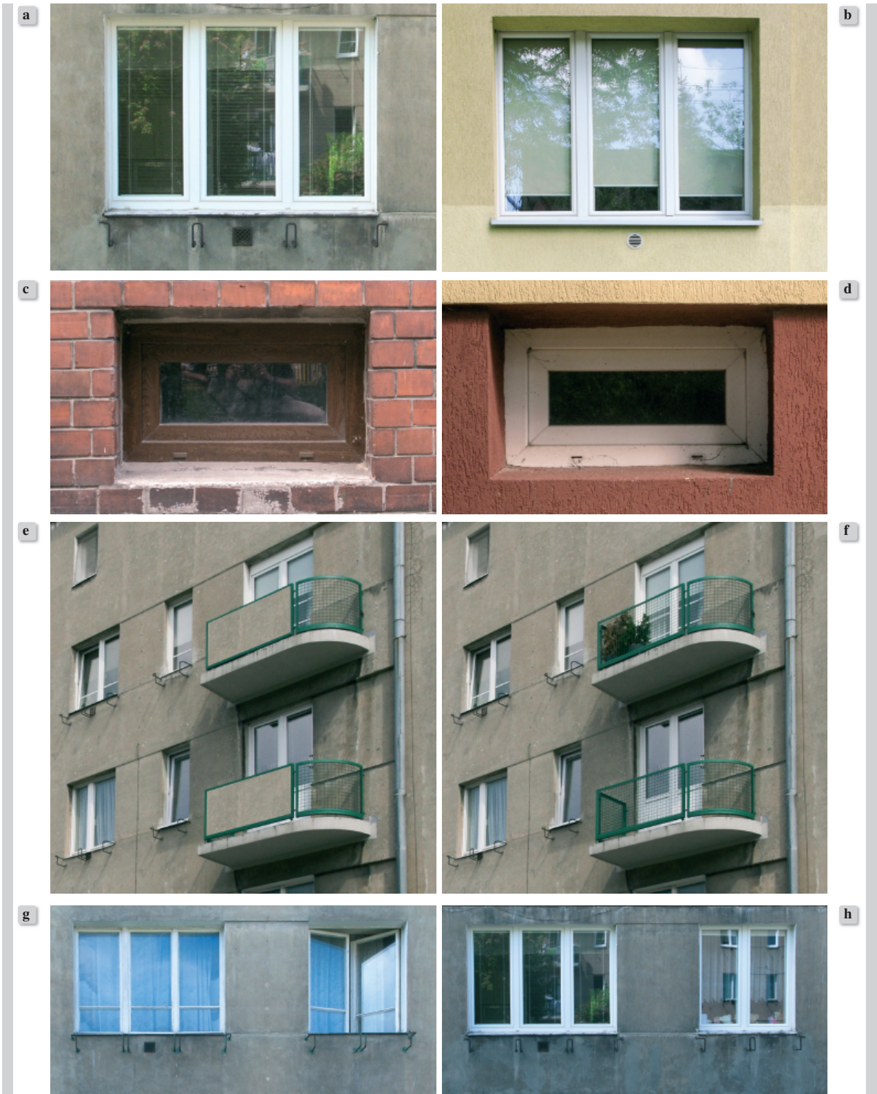
Figure 3. Examples of original and secondary design solutions from ZUS modernism housing estate in Lodz, Poland. Source: Author (2013). a) original colour and pattern of plaster; (b) secondary colour and pattern of plaster; (c) original plinths; (d) secondary plinths; (e) original balconies; (f) secondary balconies; (g) original windows subdivides; (h) secondary windows subdivides
