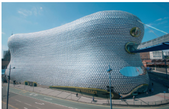
Figure 10. Selfridges in Birmingham, proj. Future Systems, 2003 [20]
