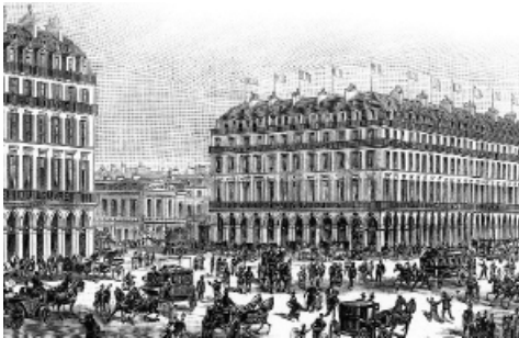
Figure 2. Grands Magasins du Louvre in Paris, [8]
