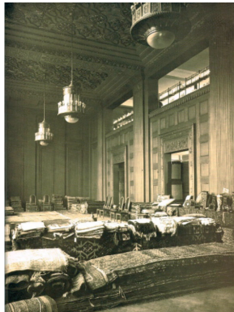
Figure 13. Department with carpets in Althoff department store, Dortmund [8]
