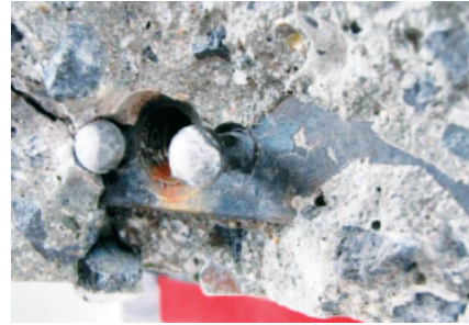
Figure 16. Failure of sleeper no. A-83/1a in static test
