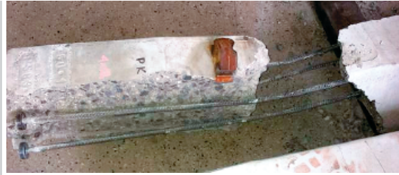
Figure 13. Failure of sleeper no. B-83/2 in dynamic test
