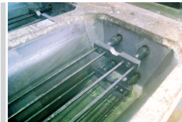
Figure 3. View of prestressing wires in "A-..." type sleepers
