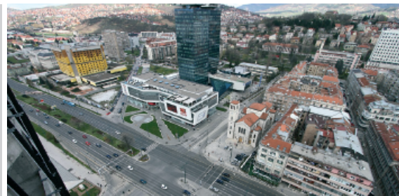
Figure 6. A clear transition between new and old structures (Source: skyscrapercity.com)
