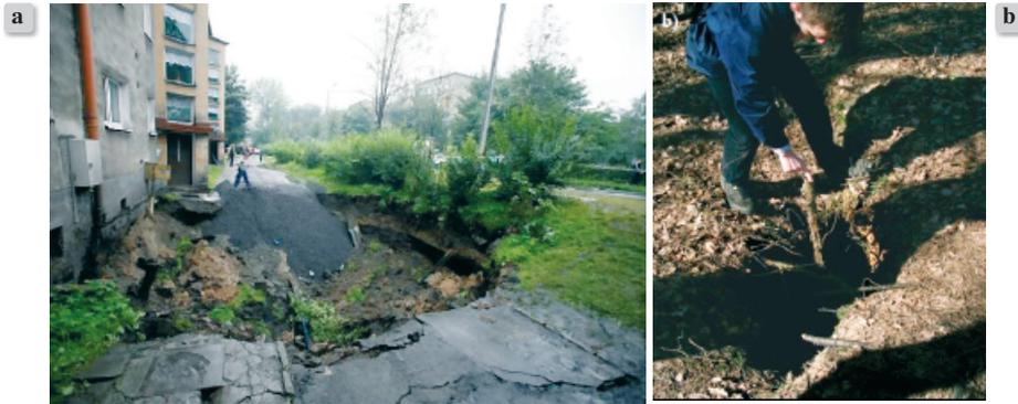
**Figure 1.** Examples of discontinuous deformations: a) local collapse (<http://bi.gazeta.pl/>), b) crevice (own archive)
