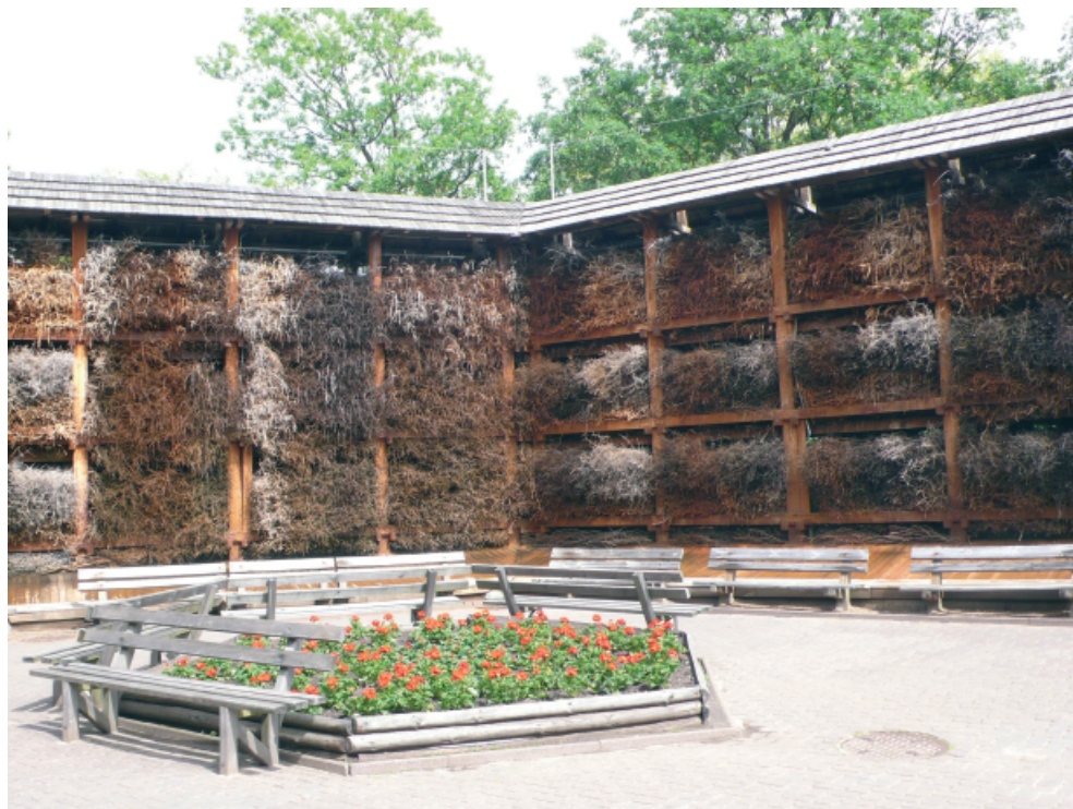
Figure 6. Spa Park in Konstancin-Jeziorna. The graduation towers were built in 1978, after the discovery of deposits of brine treatment. Source: photo by arch M. Piechotka, 2013
