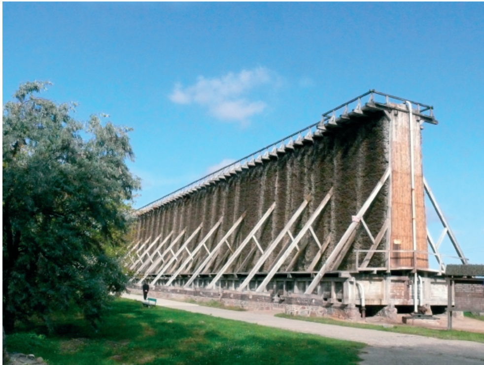
Figure 2. The Graduation Tower Spa Park in Nałęczów (one of three still existing wooden structures), designed by Jakob Graff and erected in 1824-1859. Source: photo by arch M. Piechotka, 2013
