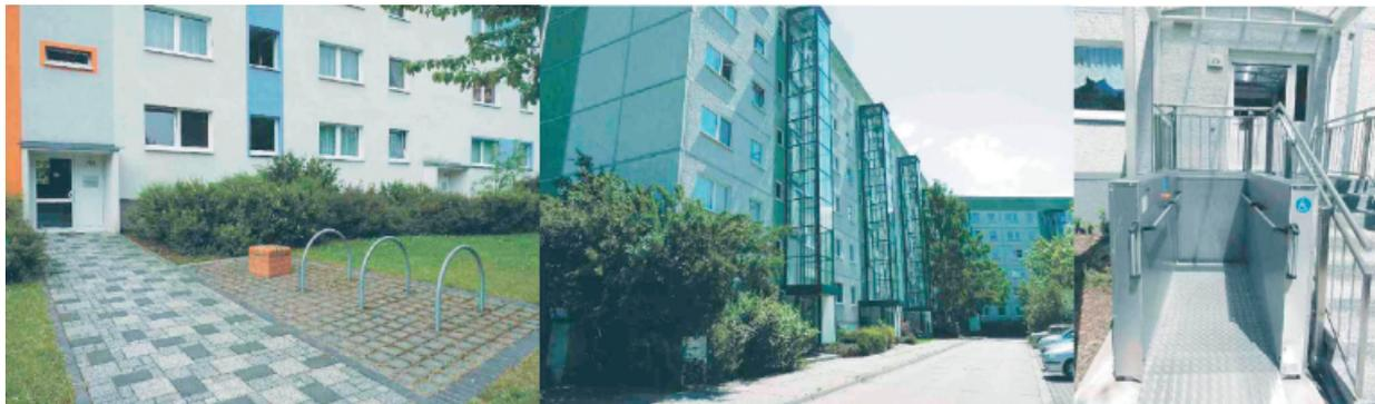
Figure 2. Liquidation of architectural barriers at Grünau Estate in Leipzig – entrance from the ground level, lifts, ramps at the exterior stairs. Source: The photograph taken by the research team
