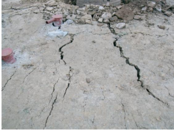
Figure 8. Ground cracking near the crater
