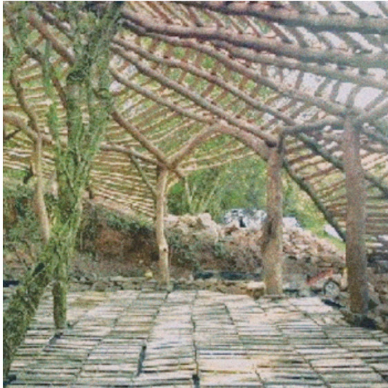
Figure 1. The skeleton of a branche house (photo [8])
