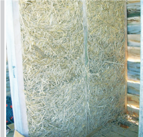
Figure 7. The wall built in a straw-clay technique (photo [12])
