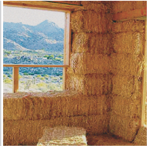
Figure 3. The wall built in a straw-bale technique (photo [11])
