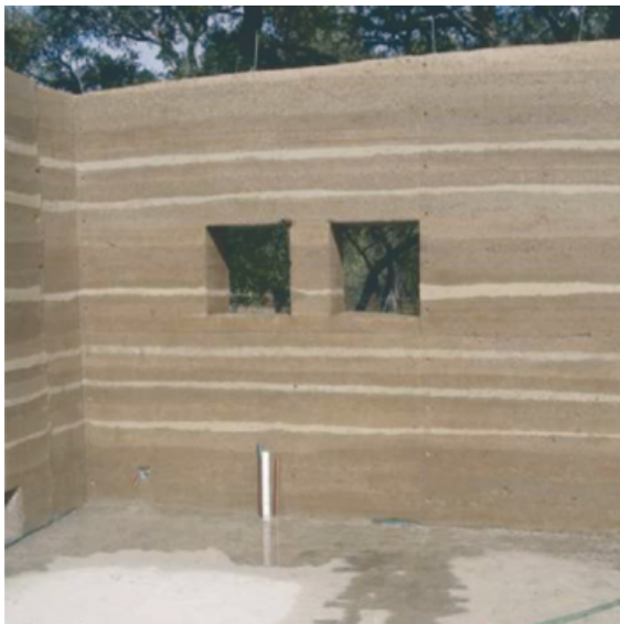
Figure 2. The wall of a building made in a rammed-earth technique (photo [5])
