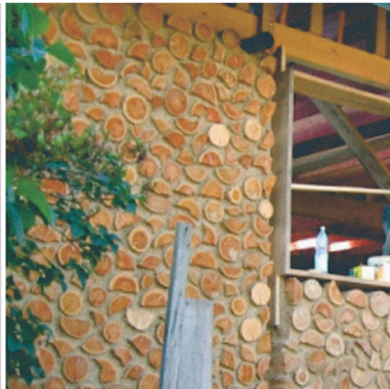
Figure 6. The wall built in a cordwood technique (photo [5])
