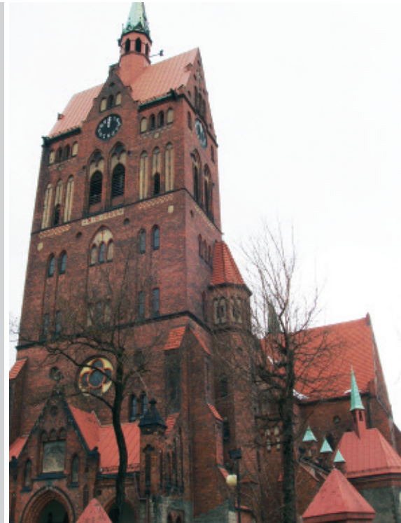
Figure 1. Saint Wawrzyniec and Antoni's church in Ruda Śląska – Wirek. South-east view
