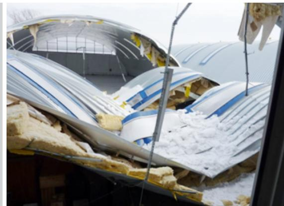
Figure 3. Arch shaped corrugated roof collapse
