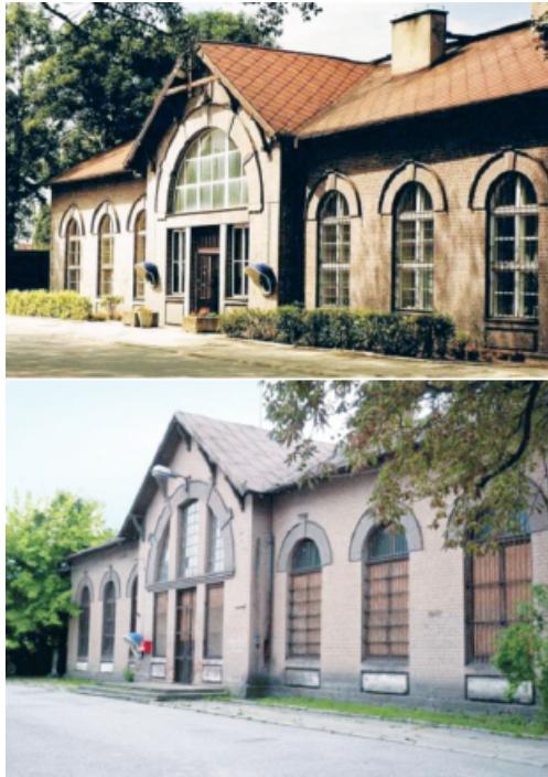
Figure 5. Railway station in Pabianice [4] and Głowno (author's photo)
