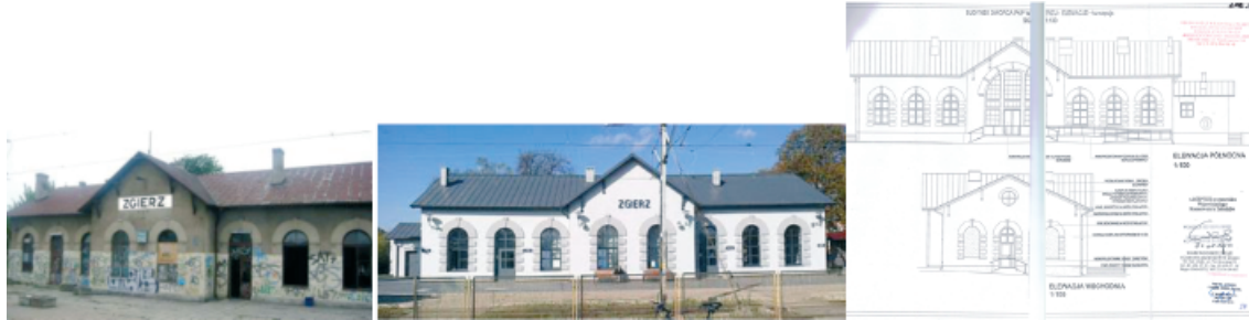
Figure 10. Zgierz railway station before and after the renovation and the documentation for the renovation of façades [5]
