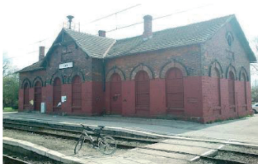
Figure 6. Railway station Łask around year 2000 before the renovation [10]
