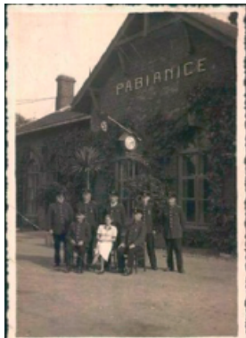
Figure 2. Railway station in Pabianice – historical picture [4]
