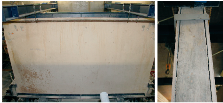
Figure 17. Plaster condition in the end of in-plane test
