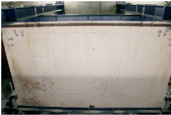
Figure 26. Crack pattern after out-of-plane test
