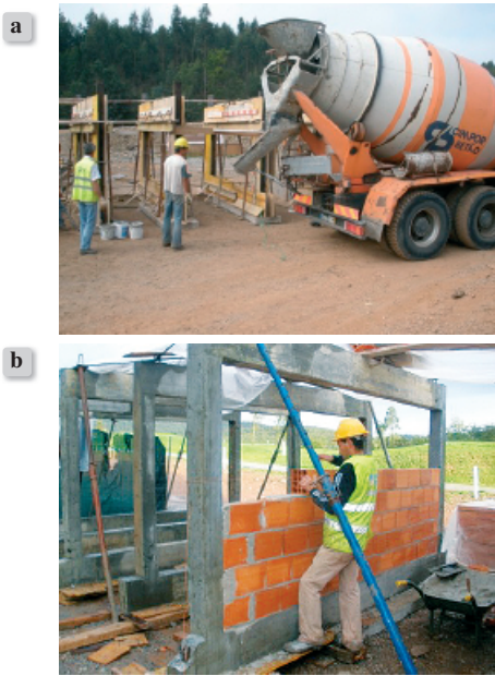
Figure 5. Construction phases of the panels: a) frame concreting; b) wall construction
