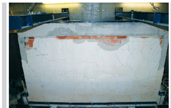
Figure 24. Crack pattern after out-of-plane test
