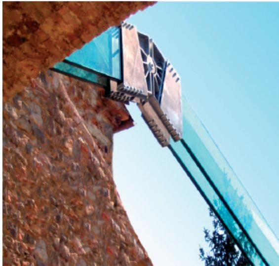
Figure 7. 6000 mm long glass beams with carbon fibre reinforcement as load-bearing elements of the saddle roof structure of “Loggia de Vicari” [5]
