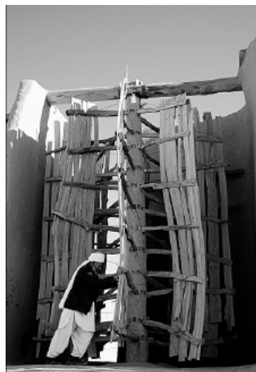
Figure 4. The wind, passing the wind catcher gate, reached the corners of eight-folded ports and moved the wheel and sails [ghader agheli]
