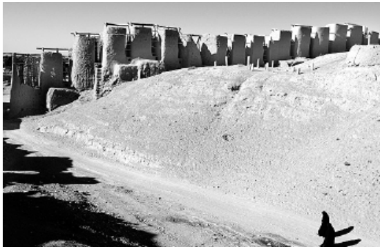
Figure 7. The Neshtifan windmills are built in a multi-storied form to exploit the wind [authors]
