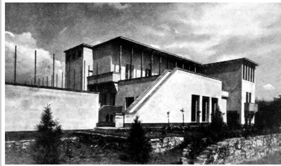
Figure 1. Zalewski's villa, garden facade, as in 1932, from: Architektura i Budownictwo , 1932, No. 8, p. 239
