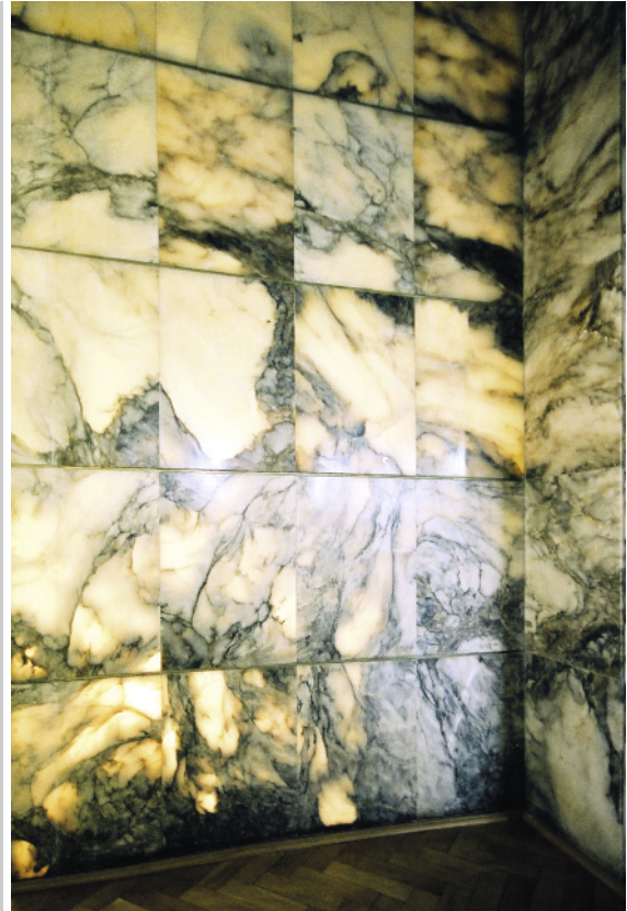
Figure 24. Urbanowicz and Muszyński's villa, alabaster screen separating the living room from the dining room at the house No. 8, as in 2006, photo by the author
