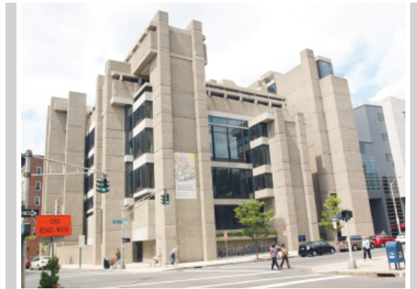
Figure 2. Yale Art and Architecture Building in New Haven, Paul Rudolph, 1958-1964 [photo: W. Niebrzydowski]
