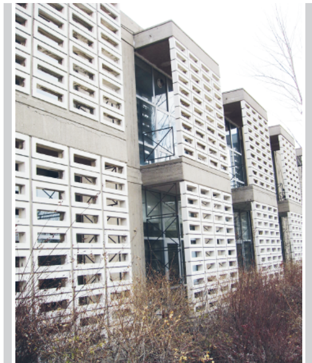
Figure 10. METU Department of Architecture Building – balconies covered by sun-breakers [photo: W. Niebrzydowski]
