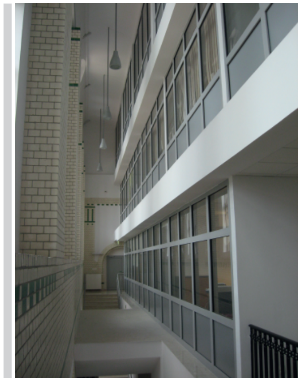
Figure 18. Interior of Machine House, currently functioning as an office building (photo J. Tymkiewicz)
