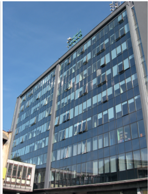
Figure 6. The back facade of “Biprohut” building in Gliwice (photo J. Tymkiewicz)
