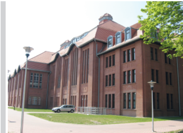
Figure 16. The old Machine House at the site of the previous coal mine in Gliwice – the back facade (photo J. Tymkiewicz)
