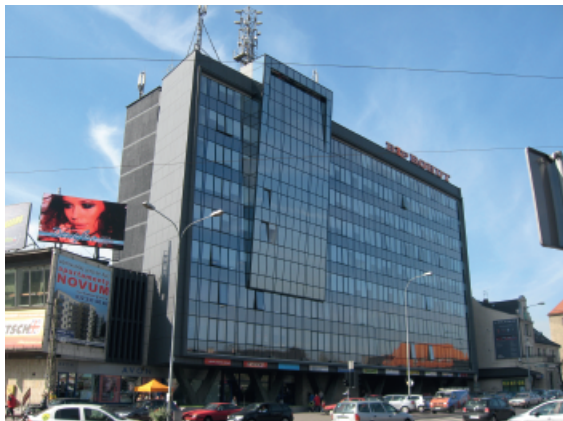
Figure 4. Replacement of glass facades – “Biprohut” building in Gliwice (photo J. Tymkiewicz)
