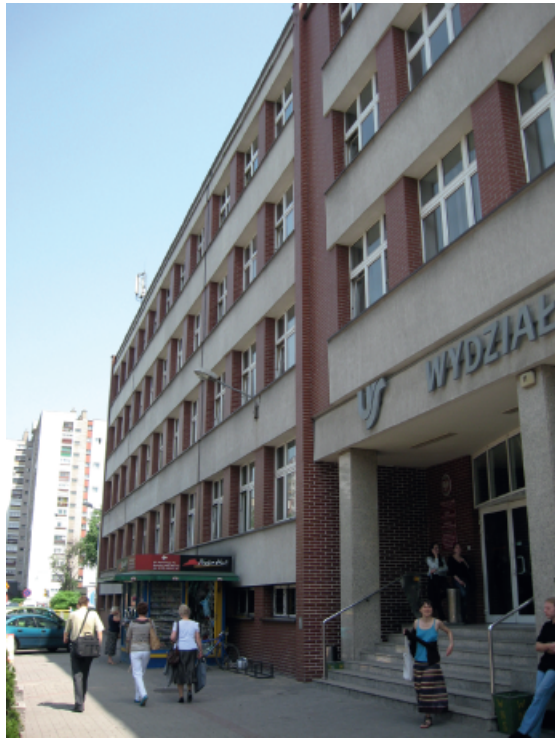
Figure 1. Faculty of Social Sciences building, University of Silesia in Katowice (photo J. Tymkiewicz)
