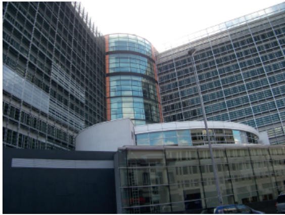
Figure 7. The headquarters of the European Commission in Brussels after modernization (photo K. Mastej)
