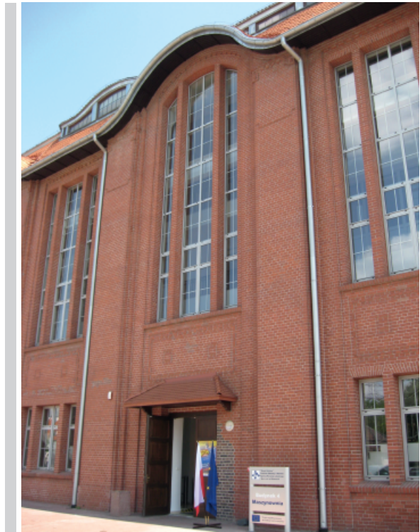
Figure 17. The entrance facade of Machine House building, Gliwice (photo J. Tymkiewicz)
