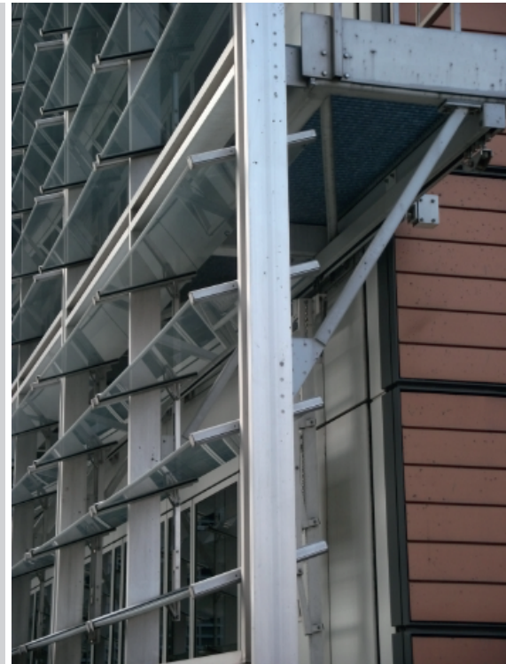
Figure 9. Details in the facade of Berlaymont building, Brussels (photo K. Mastej)
