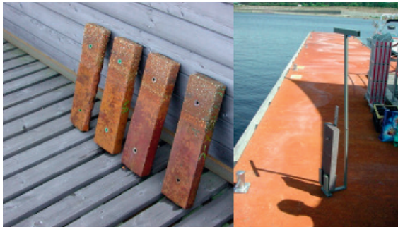
Figure 31. Samples with different concrete mix design, collected by means of a special removing assistance after a water load of one years in the lake of Partwitz
