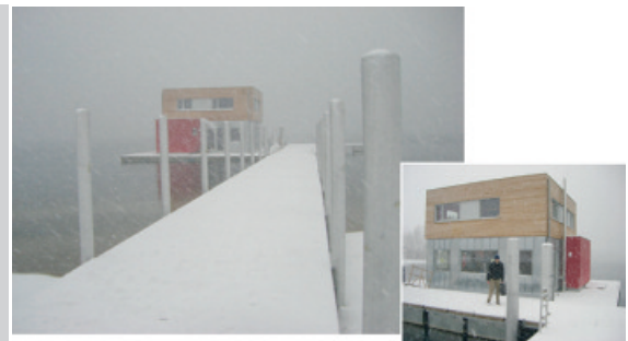
Figure 16. Floating bridges of the diving school on lake “Gräbendorfer See” during wintertime. German district Lusatia, near the border with Poland
