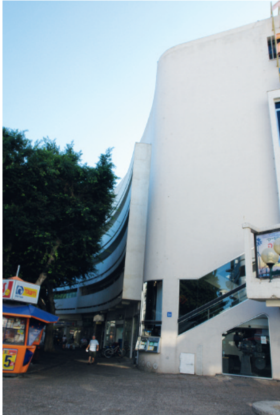
Figure 6. Arieh Sharon; Chan (Han) Cinema at Dizengoff Square, Tel Aviv, 1950. The building follows the round form of a square
