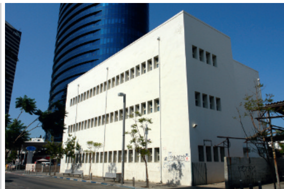
Figure 3. Erich Mendelsohn, Max Pine School for Boys, 15 Haroshet Str., Tel Aviv, 1935-36. View from the S/E. Building represents unusually simple and restrained trend, probably because of small funds available and modest location within industrial zone of the city
