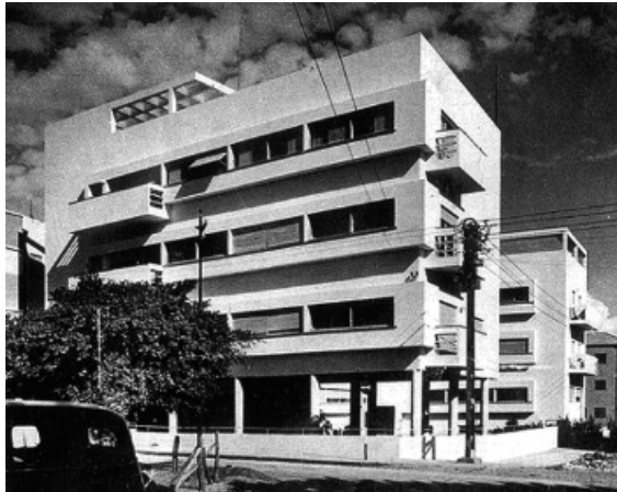
Figure 8. Ze'ew Richter, the Engel House, 84 Rothchild Blvd. The first house in Tel Aviv on the pilotis, 1933, Photo: Itzhak Kalter, www.flickr.com/photos/isotype75/393452084/
