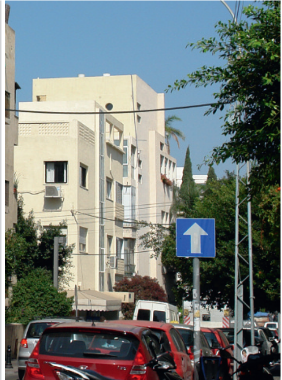
Figure 7. Shlomo Bernstein, 95 Ahad Ha'am Str., Efroni House, Tel Aviv, 1934; the use of pre-fab perforated blocks was repeated later in many houses
