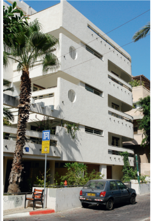
Figure 13. Lucjan Korngold, 65 Shenkin Str. This building is now considered one of the best examples of Tel Aviv architecture of the thirties
