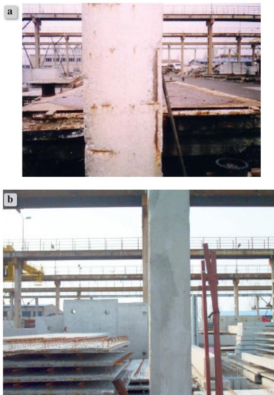
Figure 9. Reinforced concrete columnar structures: a) corroded concrete reinforcement, b) after renovation
