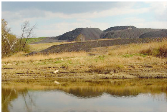
Figure 9. The “Pochwacie” dump formed now at the Zofiówka Mine covers the area of 138 ha, is 75 m high and its capacity is 123 million Mg
