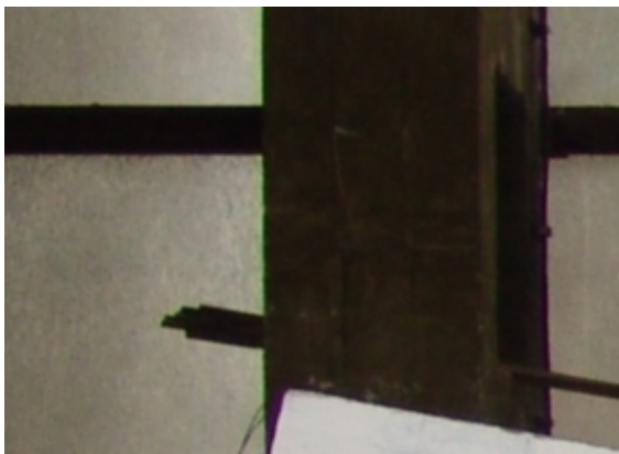
Figure 10. End-zone of slab HCS-4 (with topping) at failure
