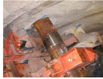
Figure 2. Curved steel pipe joints made of Iron based SMA for tunnel construction, pipe diameter 250 mm (Photo: Awaji Material)
