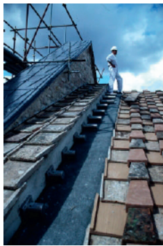
Figure 6. Back view of the historic gable (Photo: FIP Industriale)
