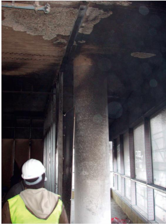
**Figure 3.** The appearance of premises after the fire – damage is clearly visible at the ceiling, while no structural damage is present in the lower part. (photo by the author)
