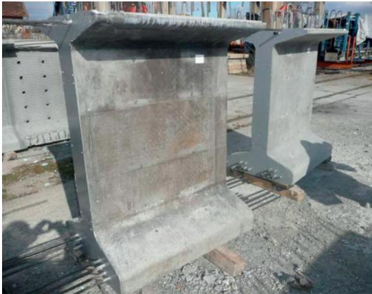
Figure 15. Segment in prestressing bed before casting and segment at the storage yard
