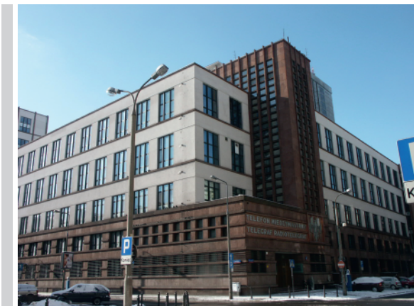
Figure 14. Arch. Julian Puterman, building of the Telecommunications Office in Warsaw, Nowogrodzka 45. Photo: author
