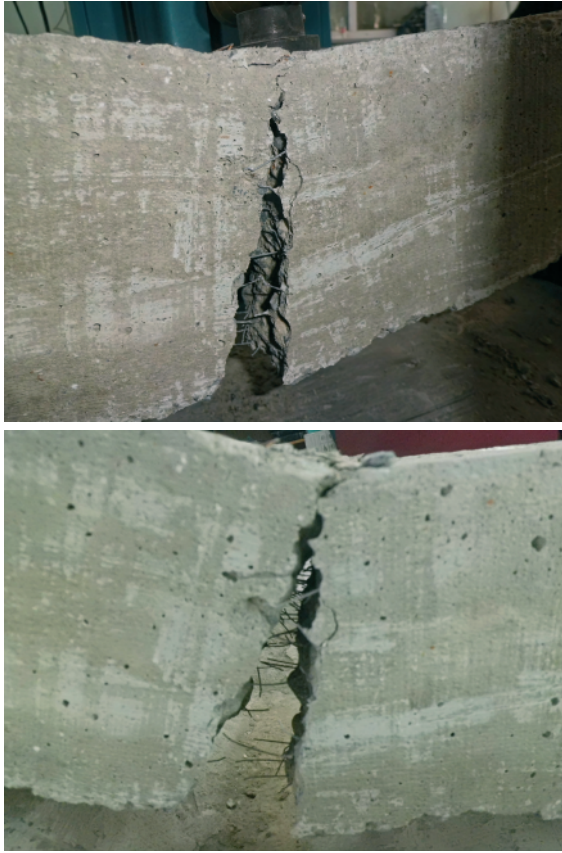
Figure 7. Improved crack growth resistance on beams specimens
