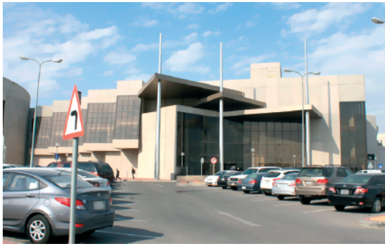
Figure 2. Exterior image of the shopping mall facility
