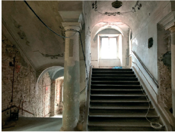
Figure 13. Żyrowa, the palace, north wing, Baroque staircase (photo by Authors)
