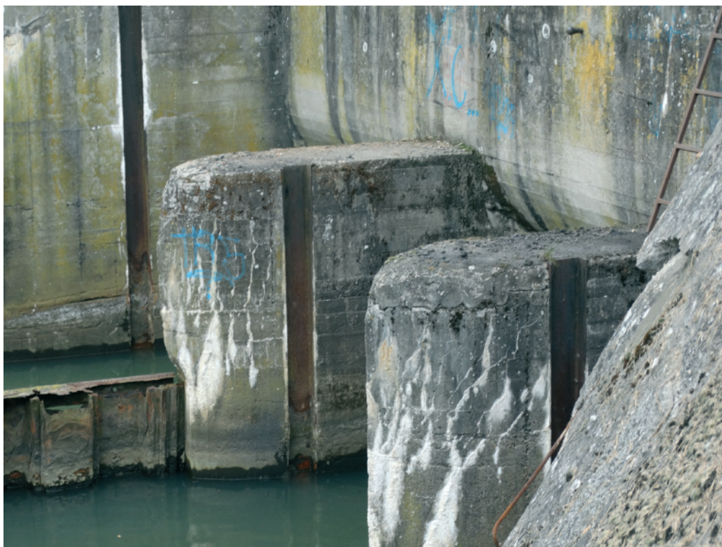
Figure 10. Destroyed surface of the concrete with the streaks of acid calcium carbonate
