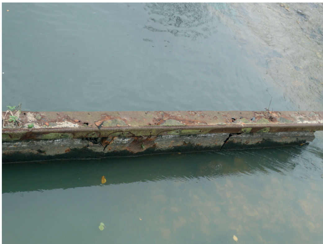
Figure 12. Bad condition of the steel sheet piles (outlet side)
