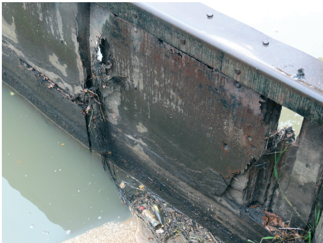
Figure 11. Strong corrosion of the steel sheet piles (inlet side)
