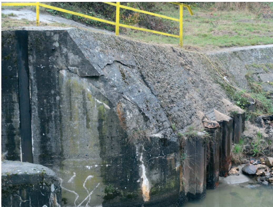
Figure 9. Destroyed surface of the concrete
