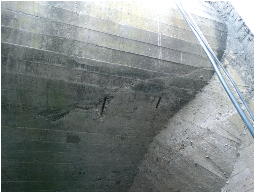
Figure 7. Damaged inlet of the duct with corroded reinforcement
